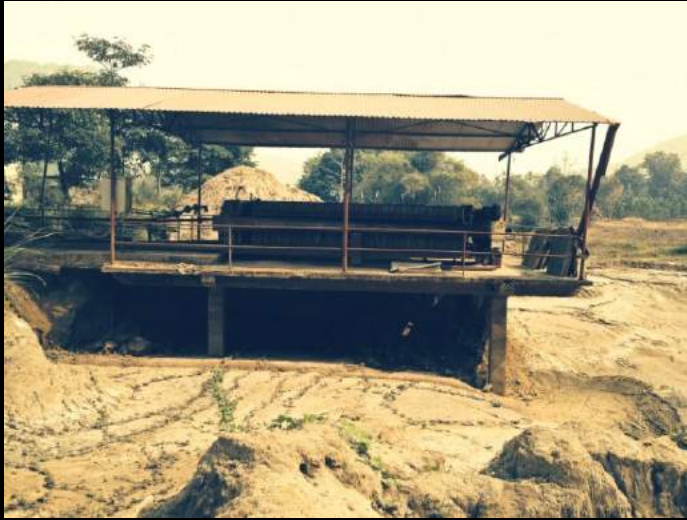
Final Filtration System – Pond Missing
