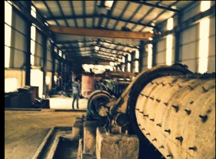
Primary Crusher, Flotation Cells and Primary Filters
