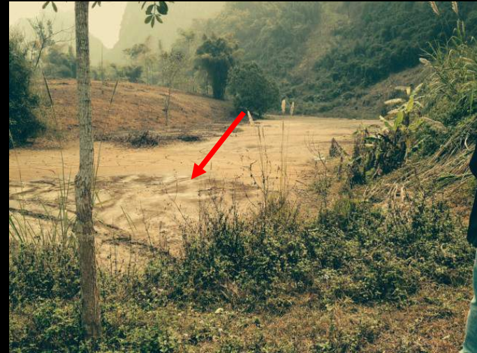
Breach in Tailings Pond Wall into Local Creek
