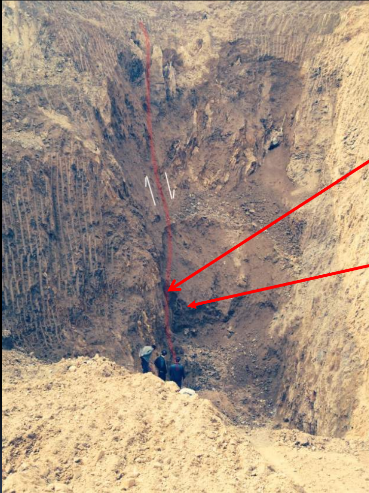
New Pit ...safety hazard!
