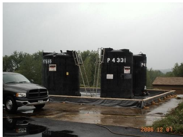
Reardon installed 22,000 gallons of storage and mixing tanks to provide a constant supply of Calcium Polysulfide for Injection Operations.
