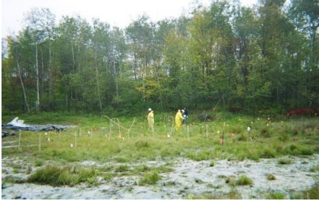
ISCO injection of Calcium Polysulfide treatment in the Lagoon Area of the site.
