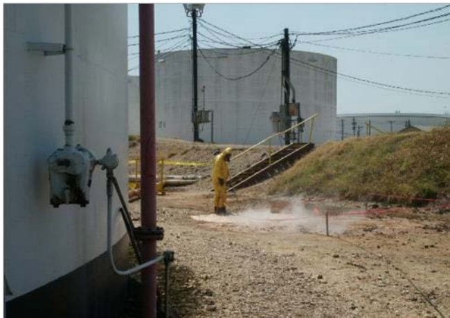
Injection of Fenton's Reagent in Tank Storage Area
