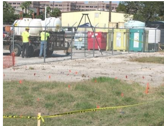
ISCO Soil Treatment Area with flagged injection points for oxidation chemical treatment.
