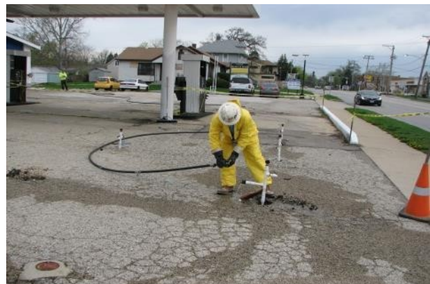
ISCO Injection of Activated Sodium Persulfate
