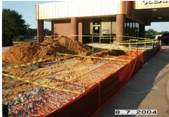
Section Exposed for Treatment of Soil
