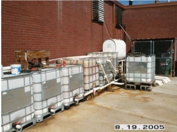
Groundwater Treatment System
