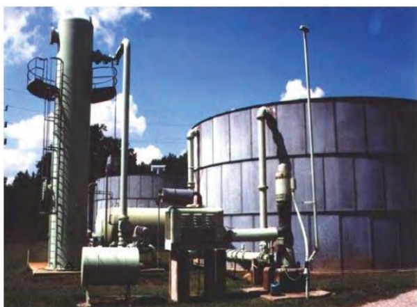
Figure 30: MUD Well and Storage Facility at FM 1960 w/ De-Gassing & De-Sanding Equipment.
