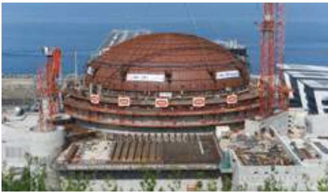
Figure E.3: Flamanville PWR plant under construction
