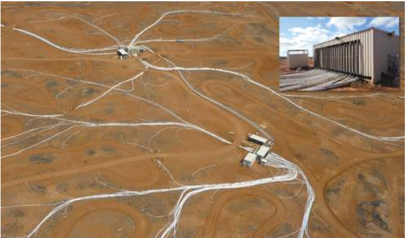
Figure 2.3: The Four Mile ISL wellfield, with inset showing pipework linking into a well-house
