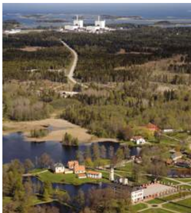
Figure I.15: Sweden's used fuel disposal facility will be located near the nuclear power plant (the white buildings shown in the background)
