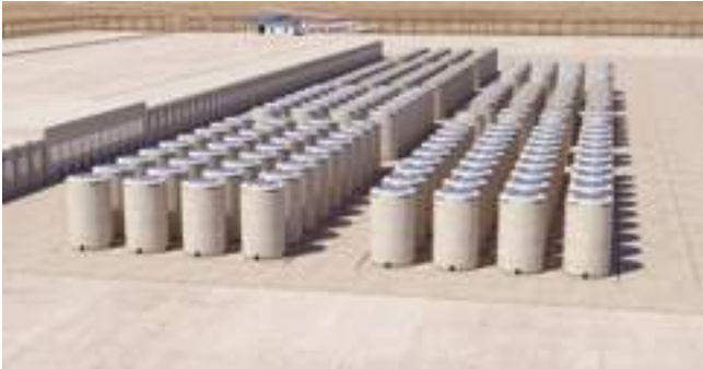
Figure 5.11: Dry cask storage facility, depicting casks stored in horizontally configured modules (left) and in a vertical configuration (centre)
